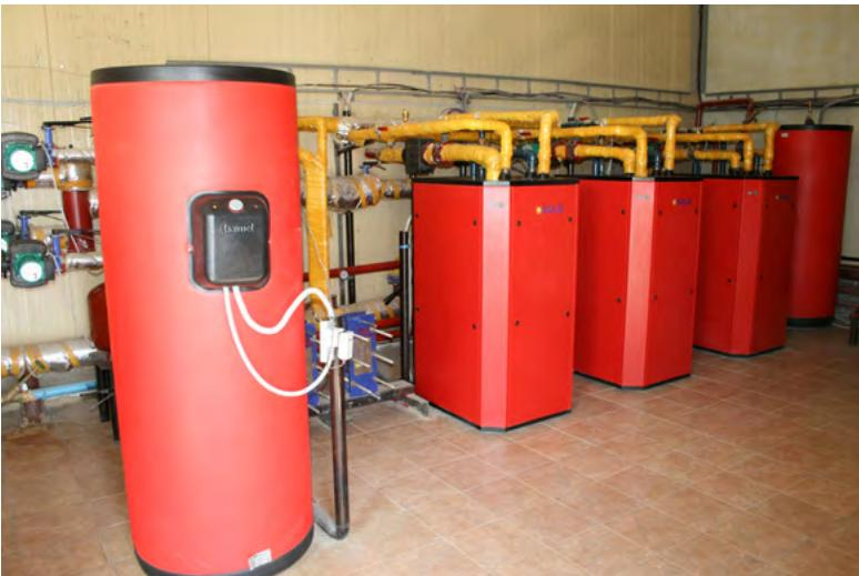
two vehicles and hot water supply (HWS) of showers and dining room for 50 seats and the administrative building of the Irkol mine. HWS operating temperature on the outlet is 55-61°C, in the return - 30-35°C. Heating system discharges the water for technological needs (hydro cleaning, container deactivation); average daily flow rate is 35-40 cubic meters. Other enterprises of Kazatomprom introduces such kind of energy-saving technology.
